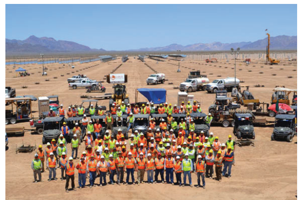
Genesis is a 250-MW solar energy project generating facility located in California's Sonoran Desert consisting of two solar electric generating facilities.
