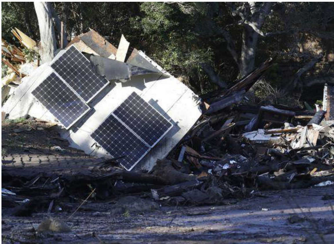
FIGURE 30 | A home with solar panels crushed in the early-2018 Montecito mudslides.
