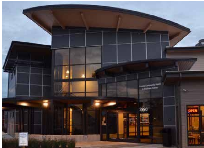
Open Door Community Health Center in Eureka, California
